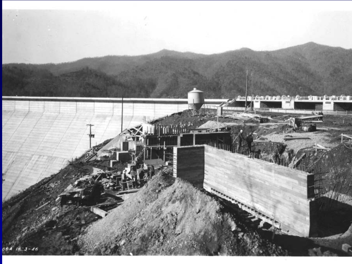
Fontana Dam Construction
