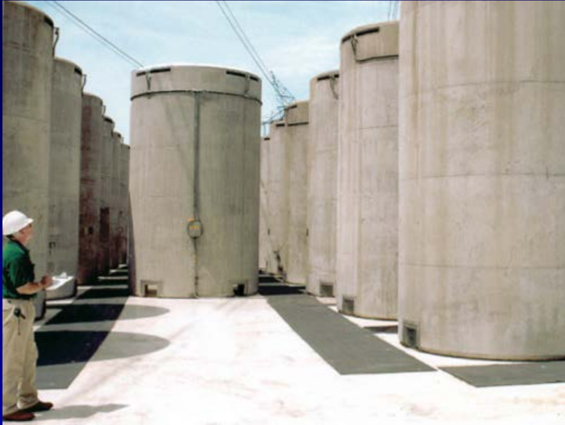
Spent Fuel Dry Cask Storage
